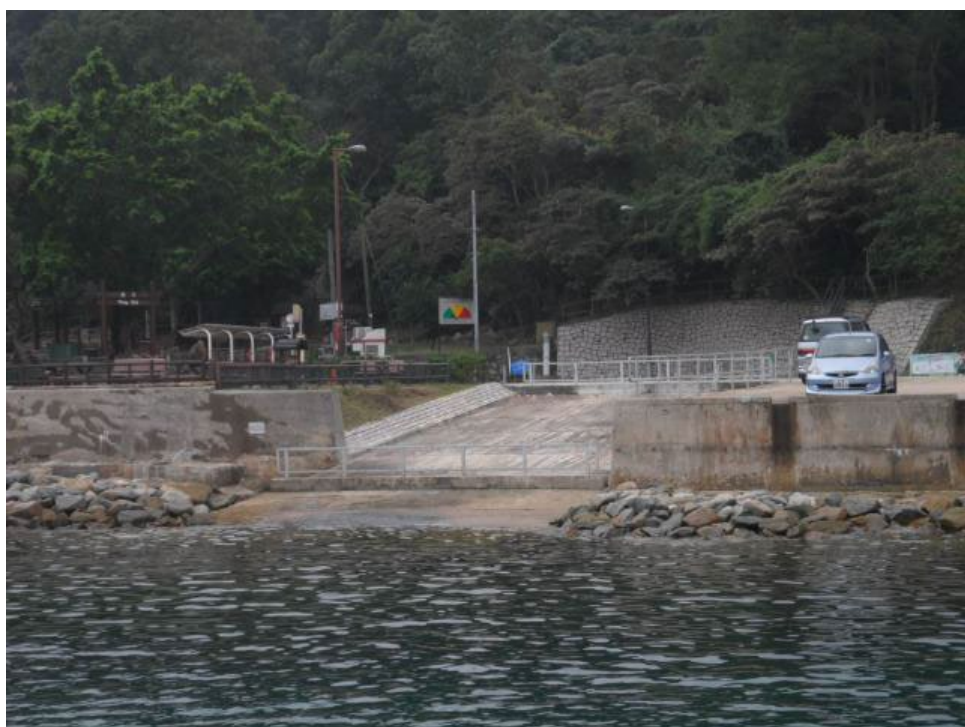
Example: Wong Shek Slipway
