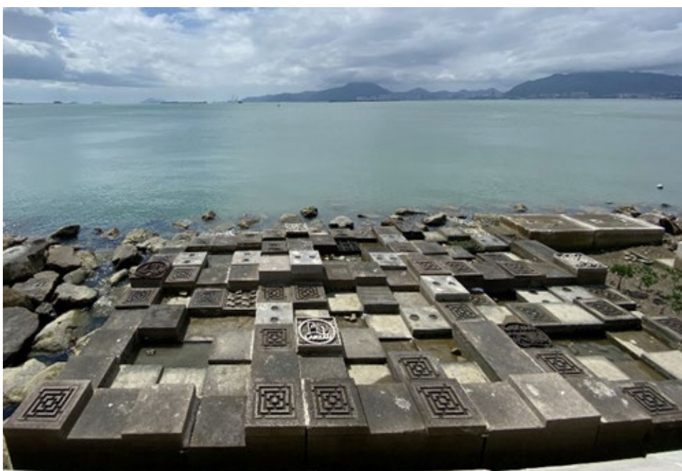
Example: Eco-shoreline at Tung Chung (bio-blocks)
